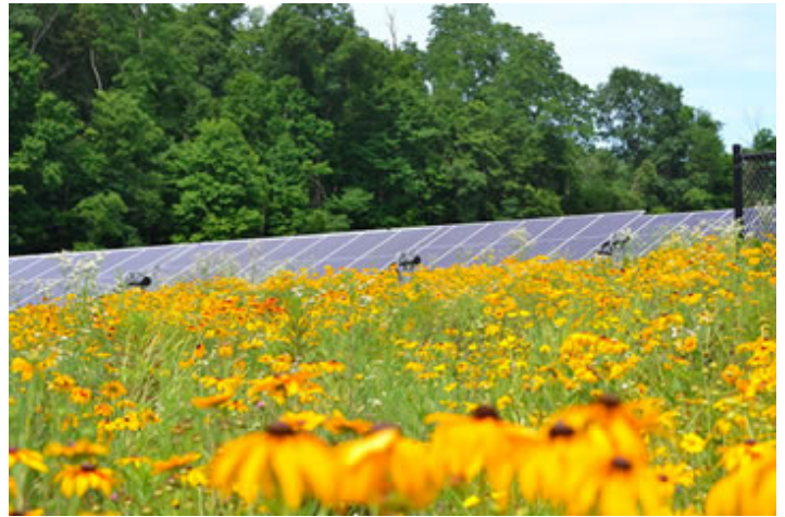
Large array site was planted as pollinator habitat – May 2018
